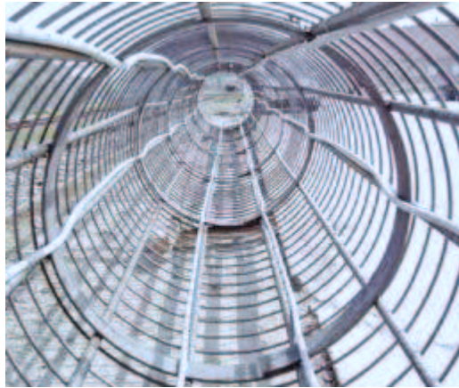
Fig.7.Geostructure (foundation pile with probes)
