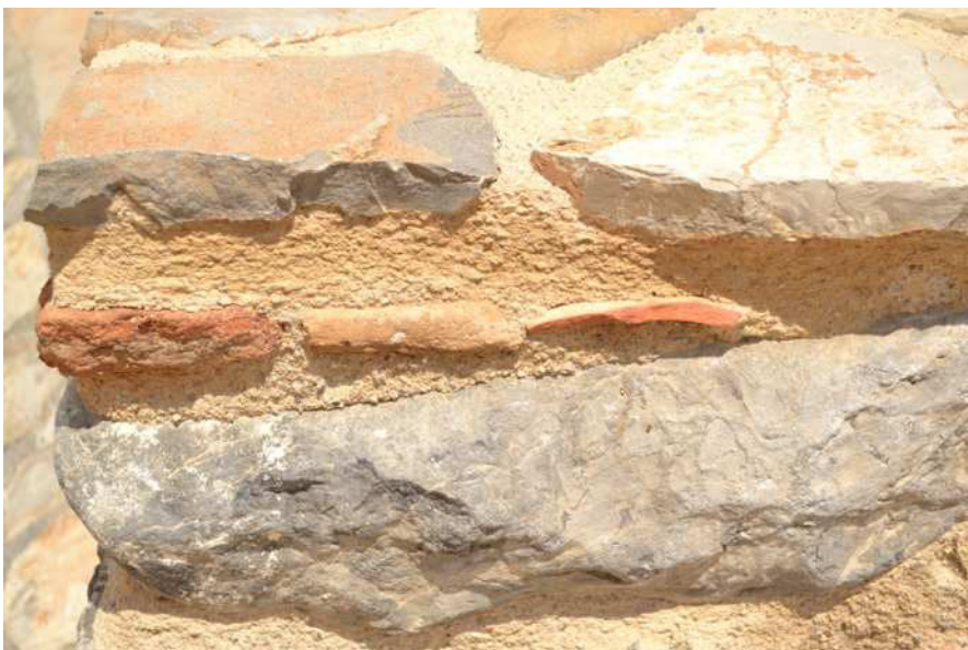
Fig. 67 Evangelismos chapel's masonry.
