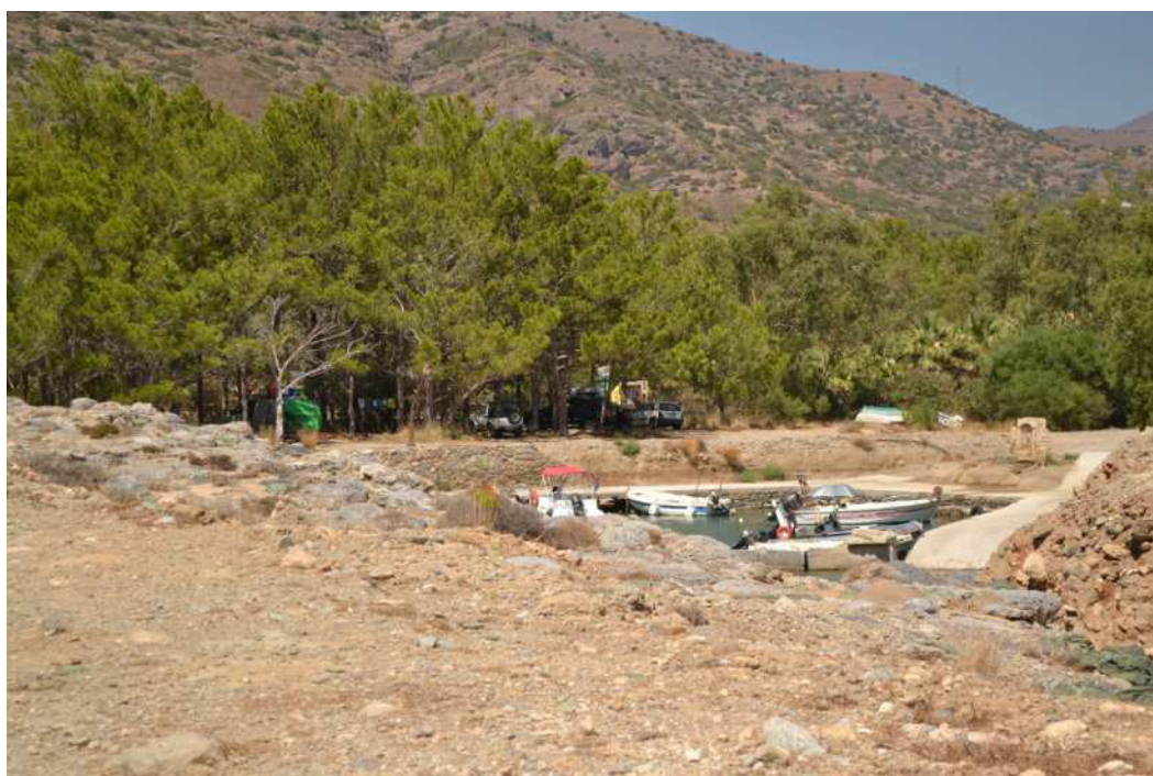
Fig. 171 The newly constructed port of Koutsouras (from N).
