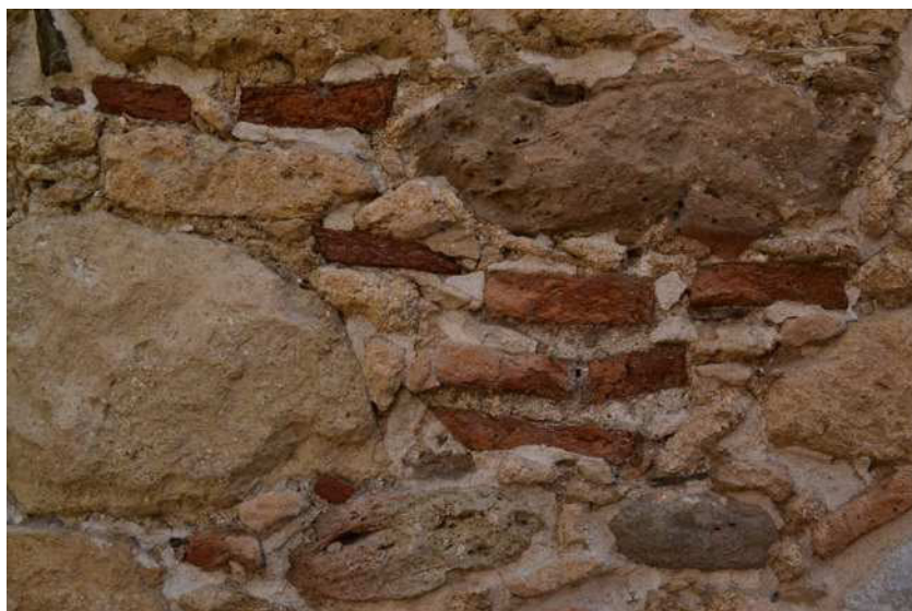
Fig. 99 Masonry of Panaghia chapel, embedded tiles.
