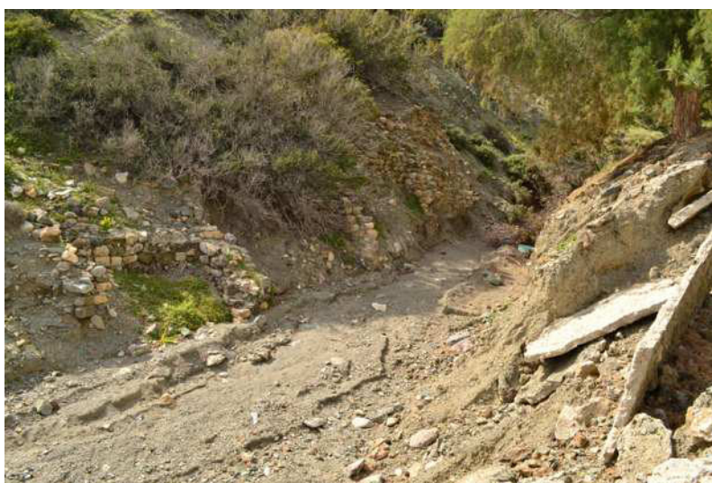
Fig. 6 Building remains in the dry stream.
