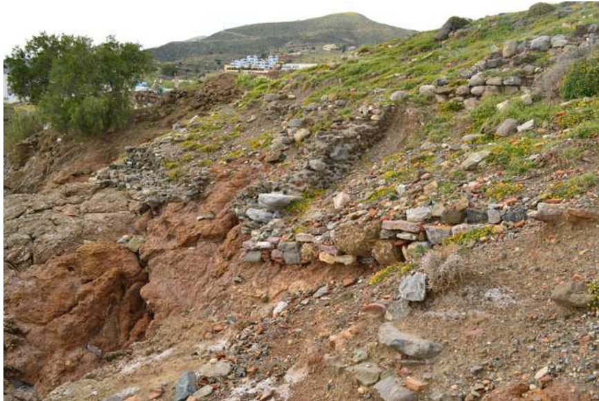
Fig. 34 Retaining walls on cape Psamidouri.
