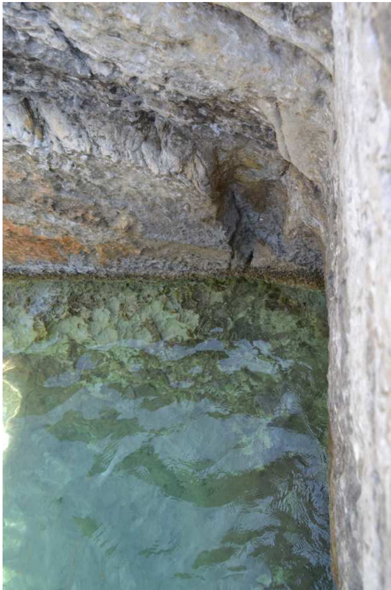
Fig. 158 Holes for the metal grid.
