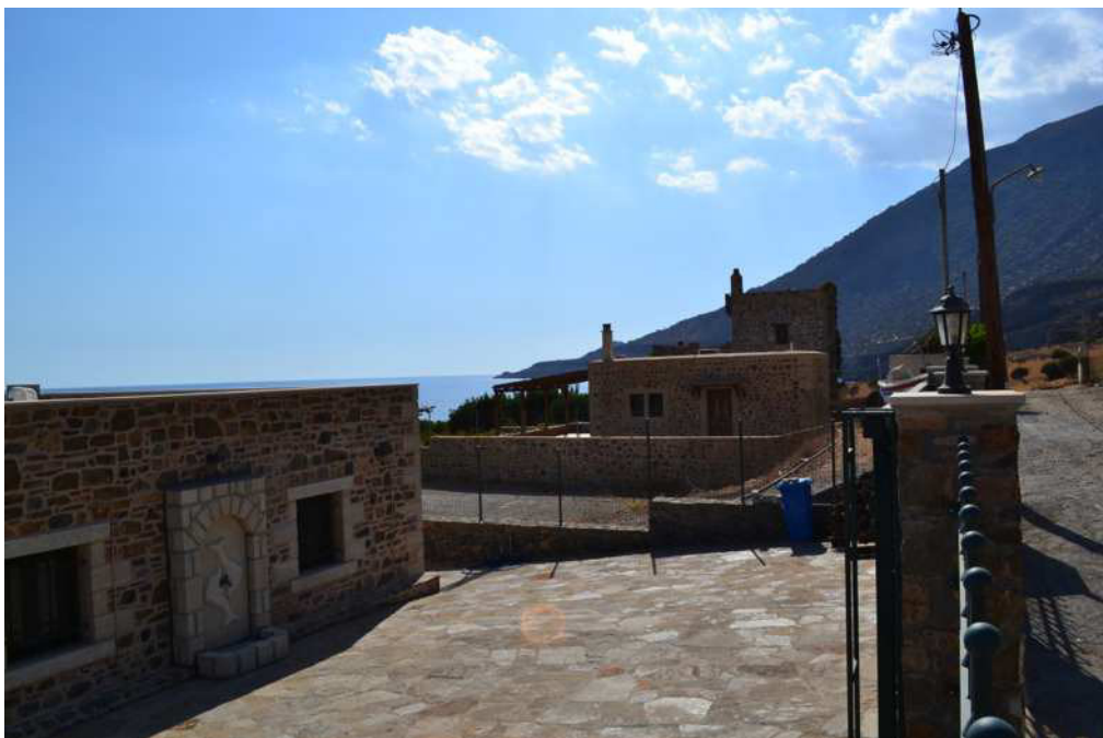
Fig. 50 Newly constructed houses at the bay of Ai Ghiannis.
