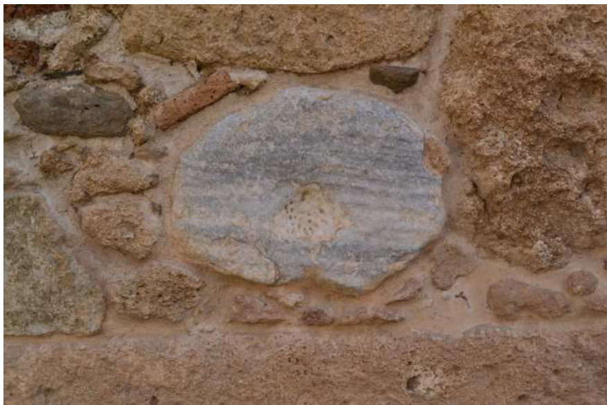
Fig. 100 Masonry of Panaghia chapel, embedded fragment of a marble column.
