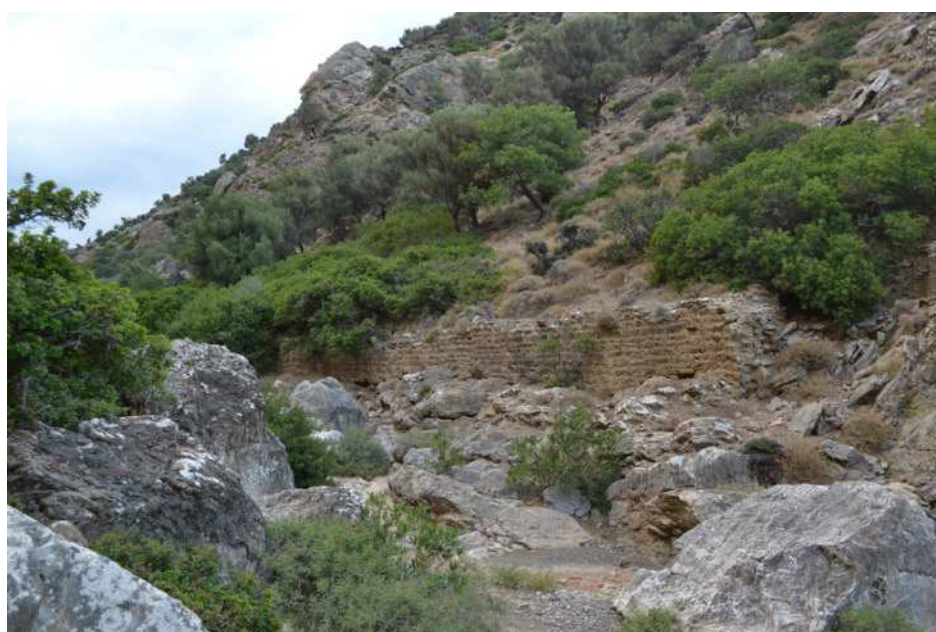
Fig. 80 Part of the Roman aqueduct in Mindris gorge
