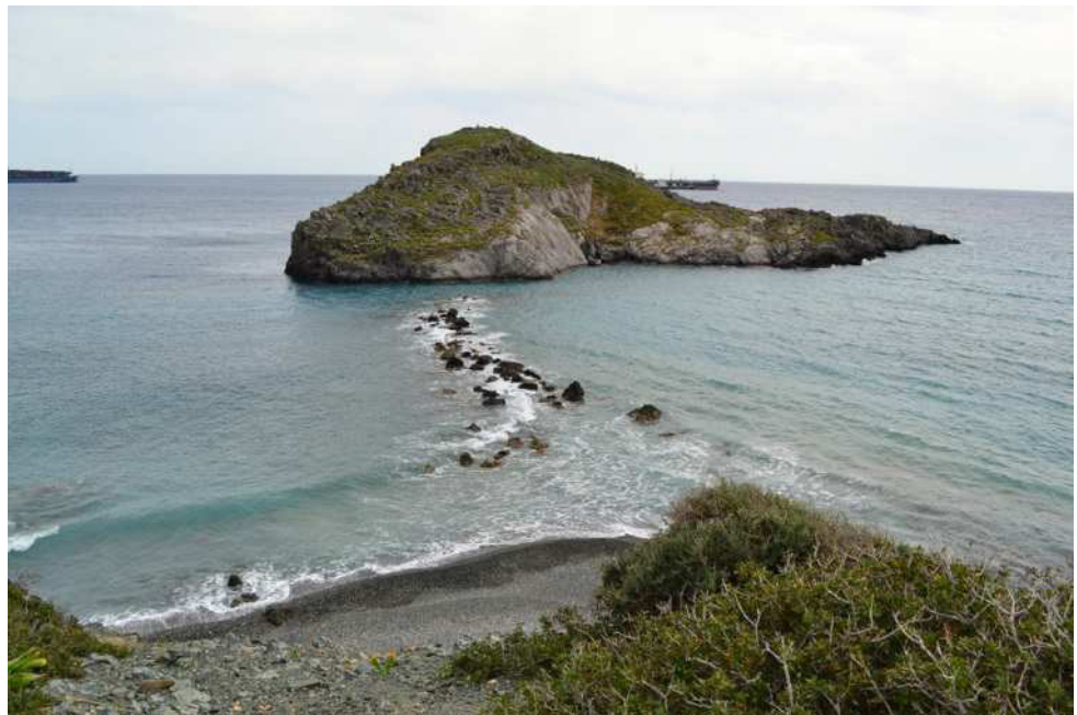
7b. The breakwater from N.
