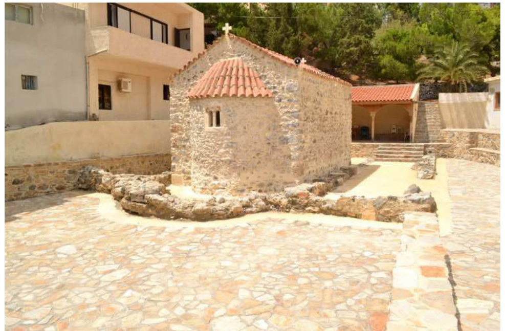
Fig. 66 Foundations of the Early Christian basilica and the 14 th century chapel of Evangelismos.
