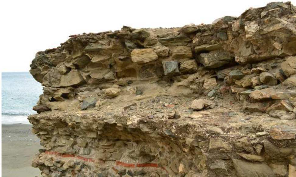
Fig. 15 Traces of the aqueduct's plastered water-channel.
