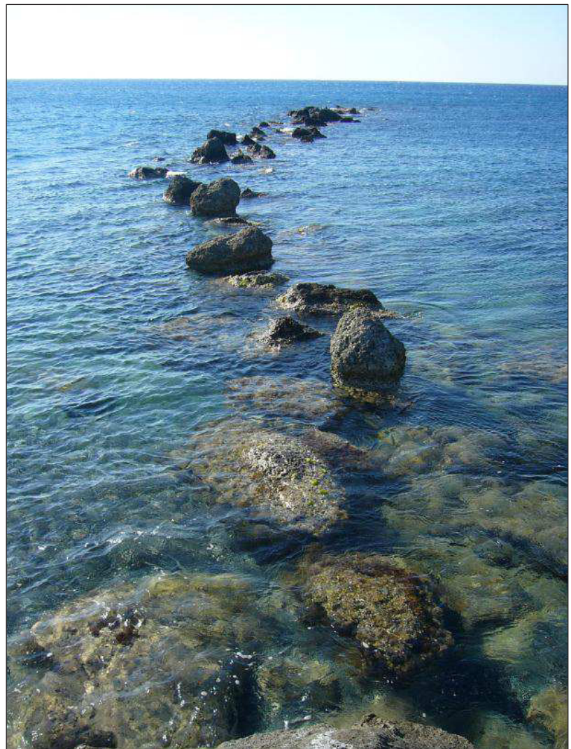
Fig. 131 Semi-submerged breakwater. (Photo source: Gallimore 2011. Photo courtesy: Scott Galimore).
