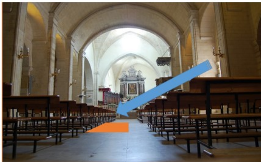
Figure 6.3 Possible air flow from the main entrance into the crypt.
