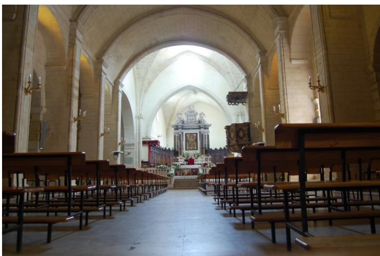
Figure 1.6. Interior view of Cattedrale Sant' Antonio Abate.
