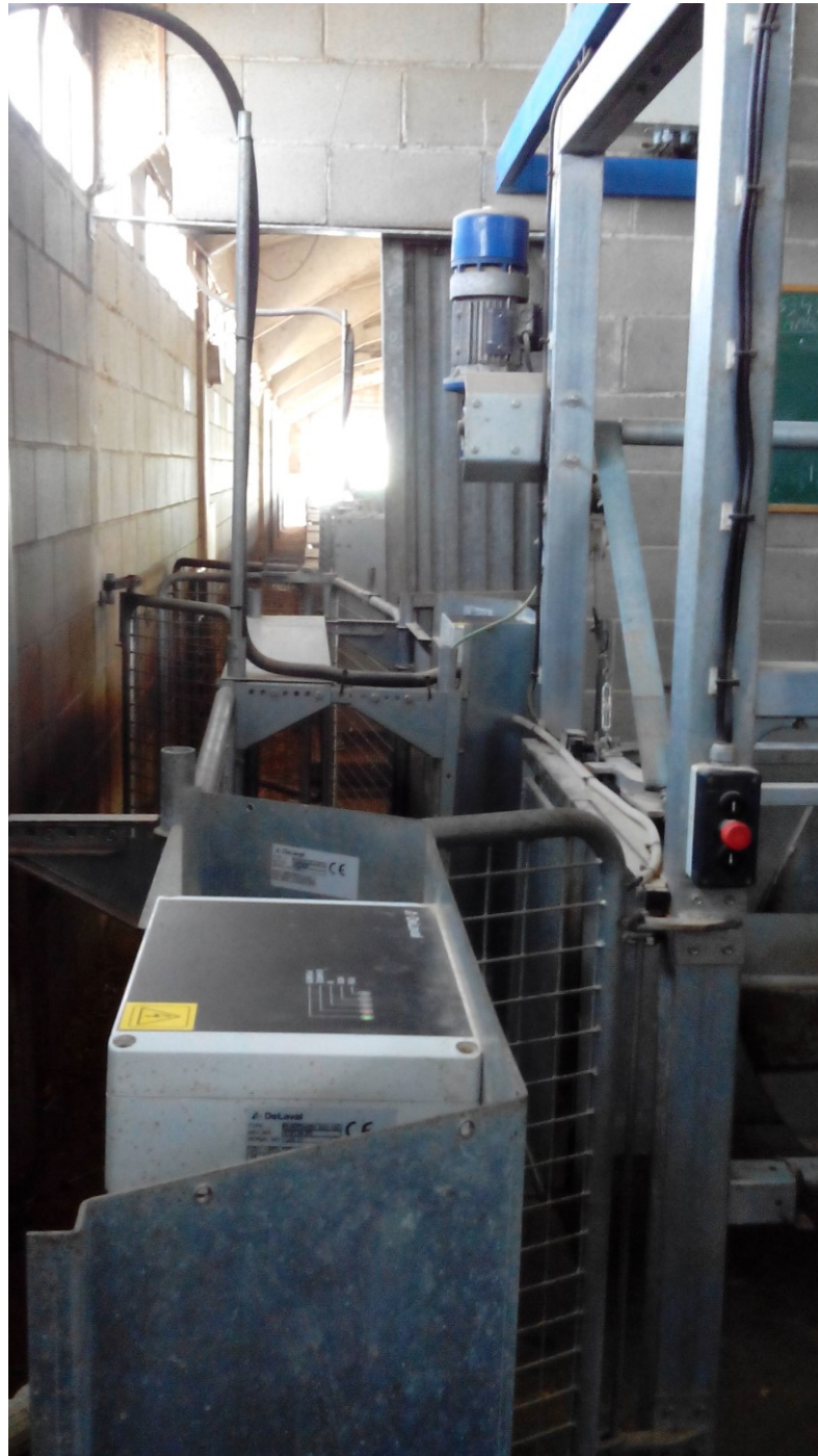
Figure 5.5. Detail electronic ID system and DeLaval sorting gate
