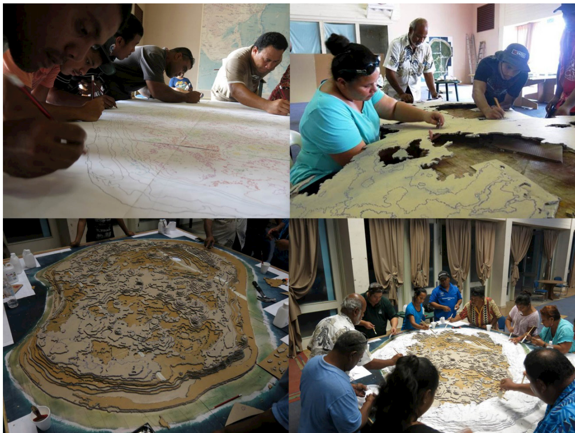
Fig. 24 People manufacturing the model; tracing, cutting, pasting layers and painting the model with white colour (they also used toilet paper between the cardboard and the paint to smooth the cardboard's edges and make the undulations of the ground more realistic)
