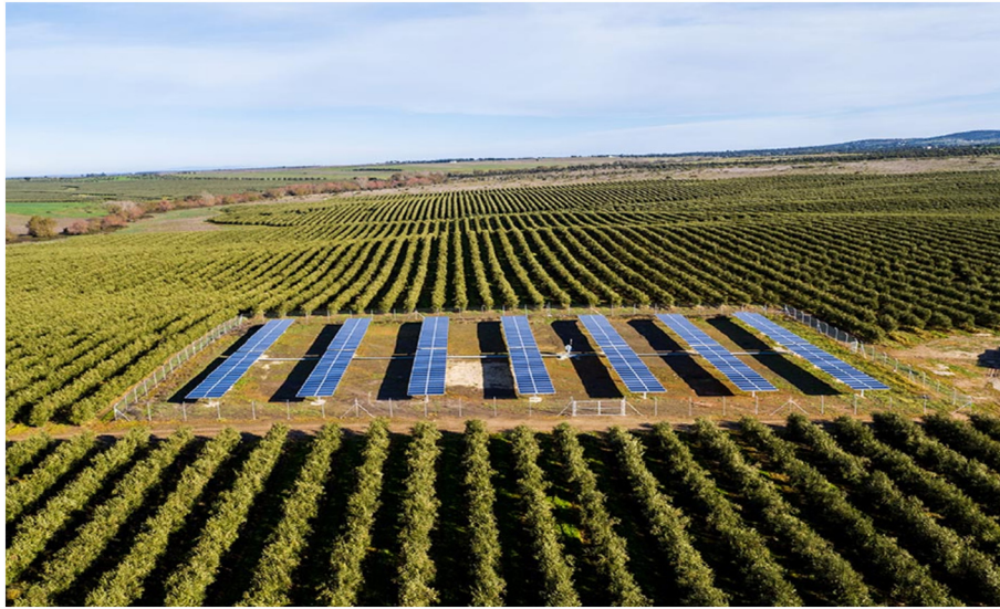
Fig. 2. Hybrid (photovoltaic + diesel) irrigation system installed in Alter do Chao (Alentejo, Portugal).
