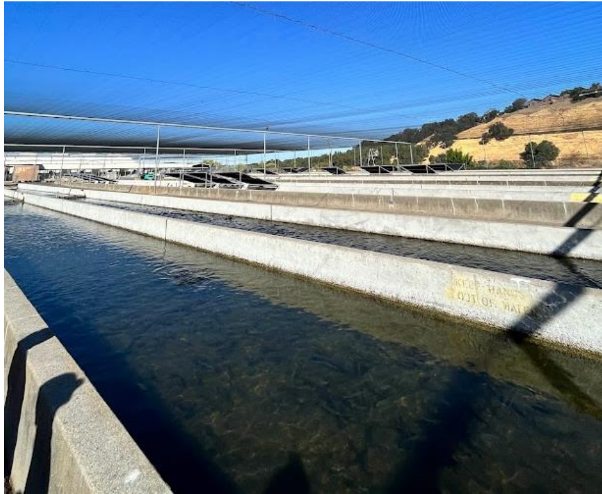
Figure 16. A flow through raceway for trout production at Sacramento State Aquatic Center. (personal picture)
