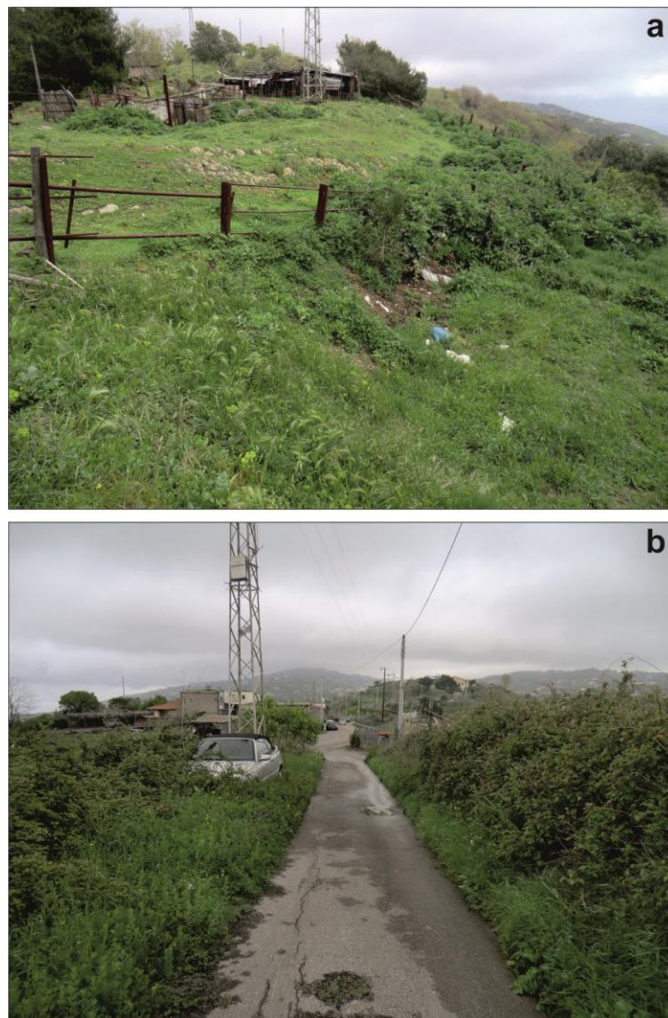
Figure 6.1 View of the crown zone; a) typical landslide terrace; b) cracks on the paved road
