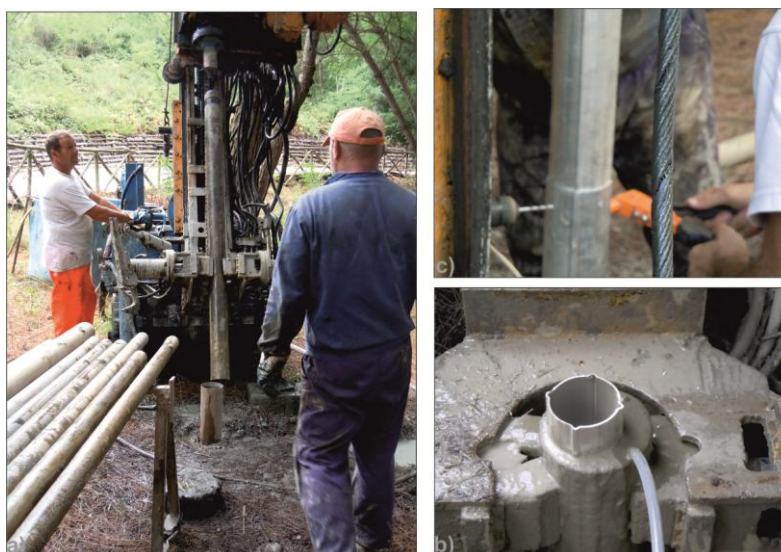
Figure 5.4 Inclinometers installation in the studied area.
