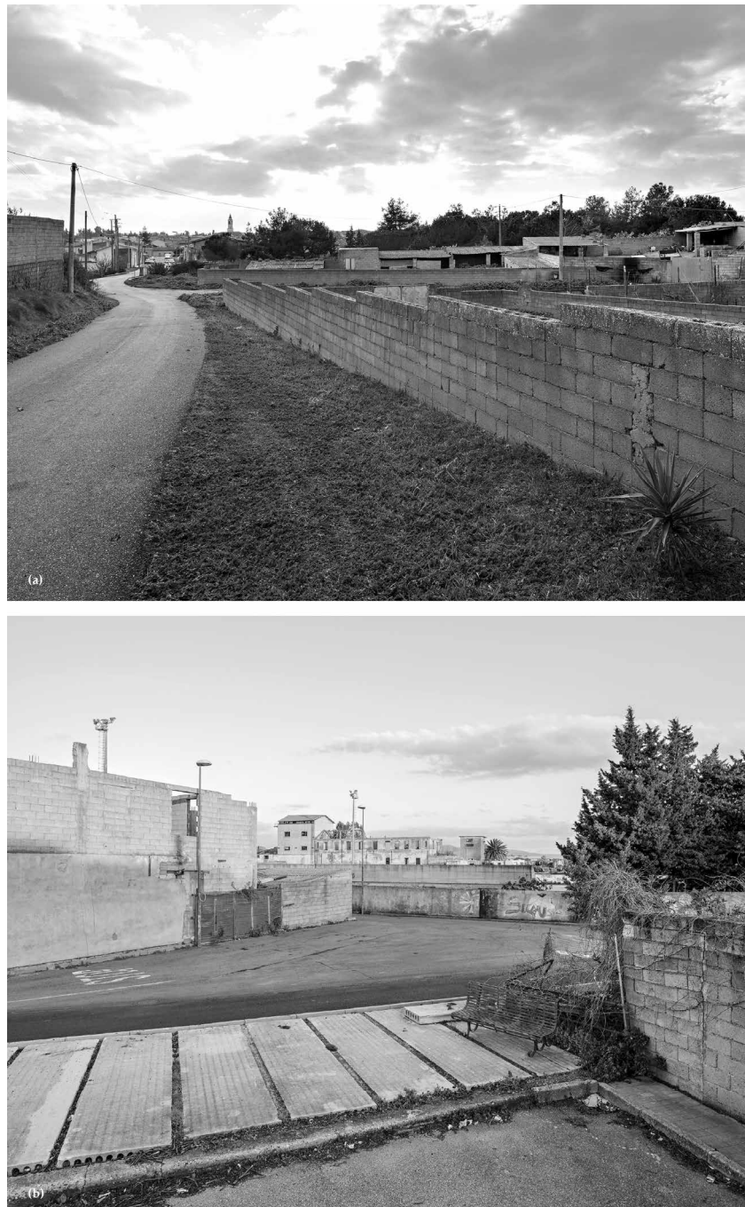
Figure 14. Incompleteness and fragmentation of the urban edge of Solarussa. (a) North urban edge of Solarussa; (b) culvert of Nura e Craba channel. Photo by D. Virdis.
